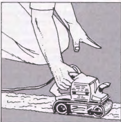
3. Sand glued joints smooth.
